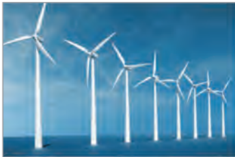
Wind power generation
