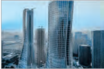
Building water supply
